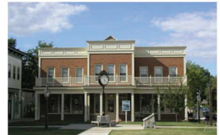
Architectural detailing- material, windows, cornice (DC, EC)
