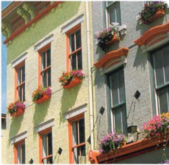
Architectural detailing- double hung windows, plantings on buildings, colors, cornice (DC, EC)
