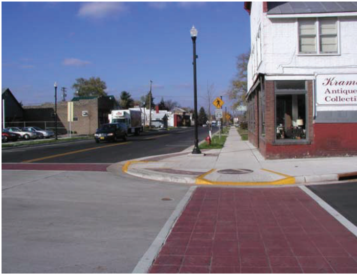
Bump Out with Special Pavement Crosswalk
