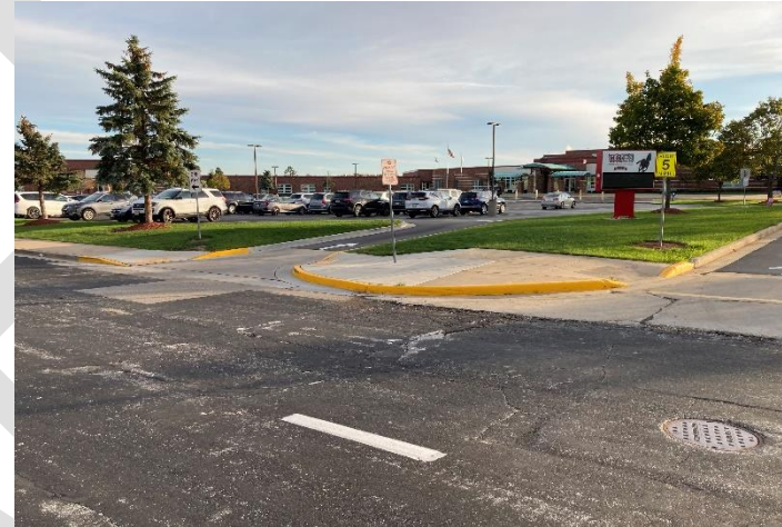
Milldrum St. along Union Grove Elementary School is scheduled for pavement replacement and utility work in 2022.
